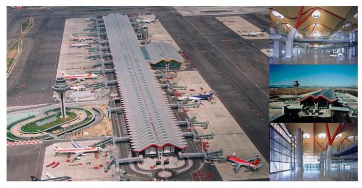
The 70,000 m2 occupied by the Satellite Building of the new terminal of Barajas Airport are distributed between a central zone of 144,00 x 180,00 m on plan and two lateral dike-like constructions of 396,00 x 54,00 m. Depending on the area, these dike-like constructions have up to three underground levels and two over ground ones. A distinctive feature of one of these dike-like constructions is its resting on the tunnel of the M-111 motorway.
